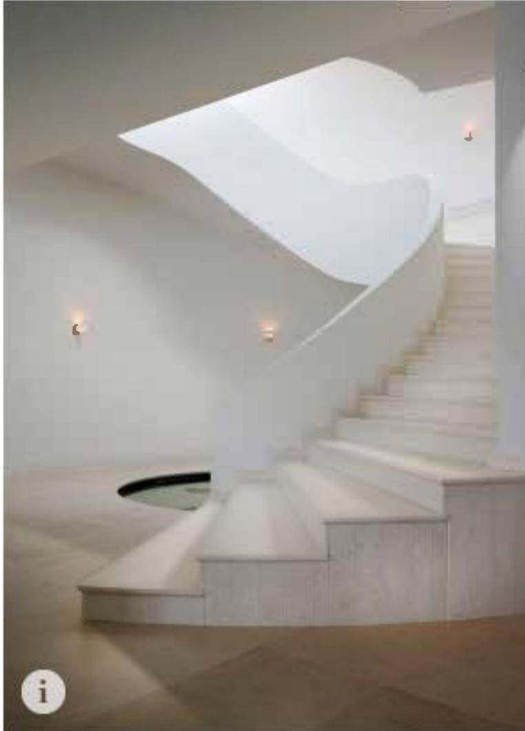
The ground floor is arranged as a series of open rooms. Guests are greeted by a grand staircase, located at the center of the house, which reaches all the way up to the roof. The stair has an outside diameter of 29 feet, and is topped by a large, glass skylight. "The width of the stair at the ground floor is nine feet, becoming gradually smaller as it spirals up to the roof terrace," Prio-Touzet says, adding that the skylight keeps the ground floor constantly illuminated during the day.
